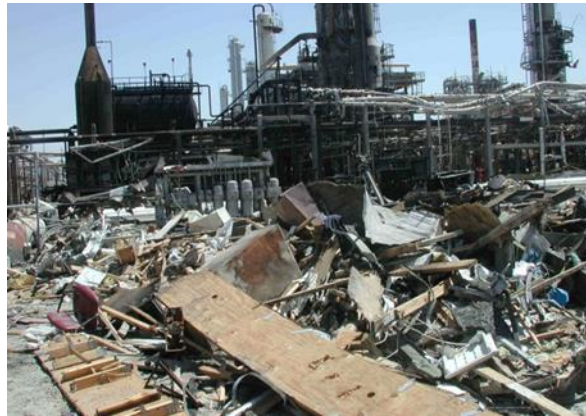
Figure 6 BPTM refinery in Texas City after the explosion
